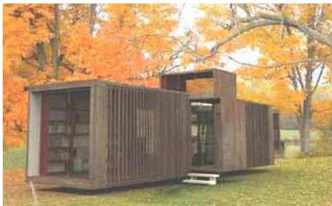
Drop House de D3 Architectes
