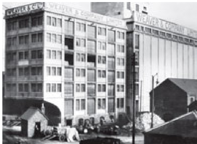
Designed by Hennebique, the Weaver & Co mill (1898) in Swansea was the first entirely reinforced concrete fully-framed building to be erected in Britain
