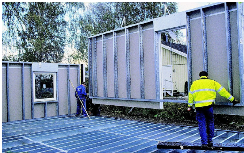
Large Pre-Fabricated Wall Panel, Lindab, Sweden
