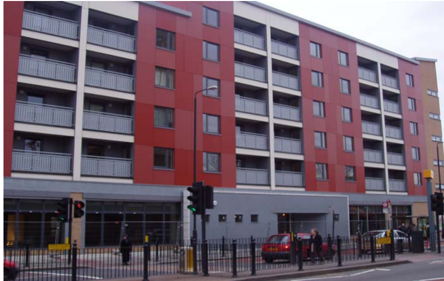
Completed Building with Offices at Ground Floor
