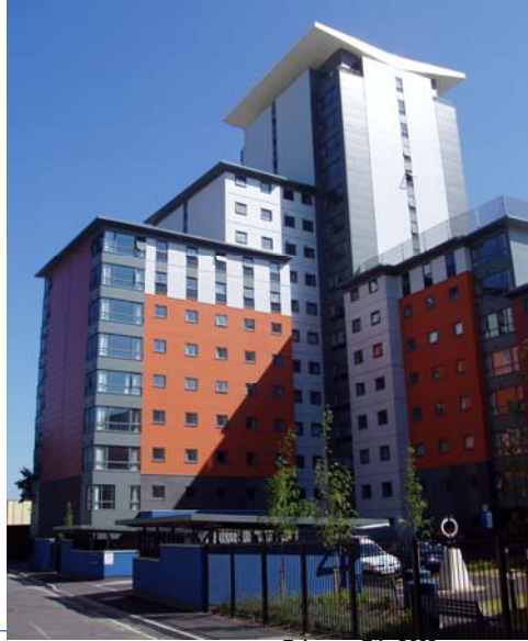
17 Storey Residential Building in Slimdek
