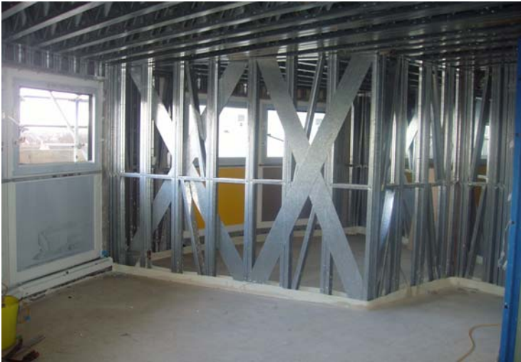
X Braced panels using Light Steel Framing
