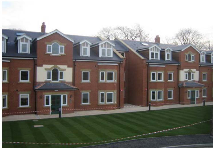
Completed building in light steel framing, Middlesborough
