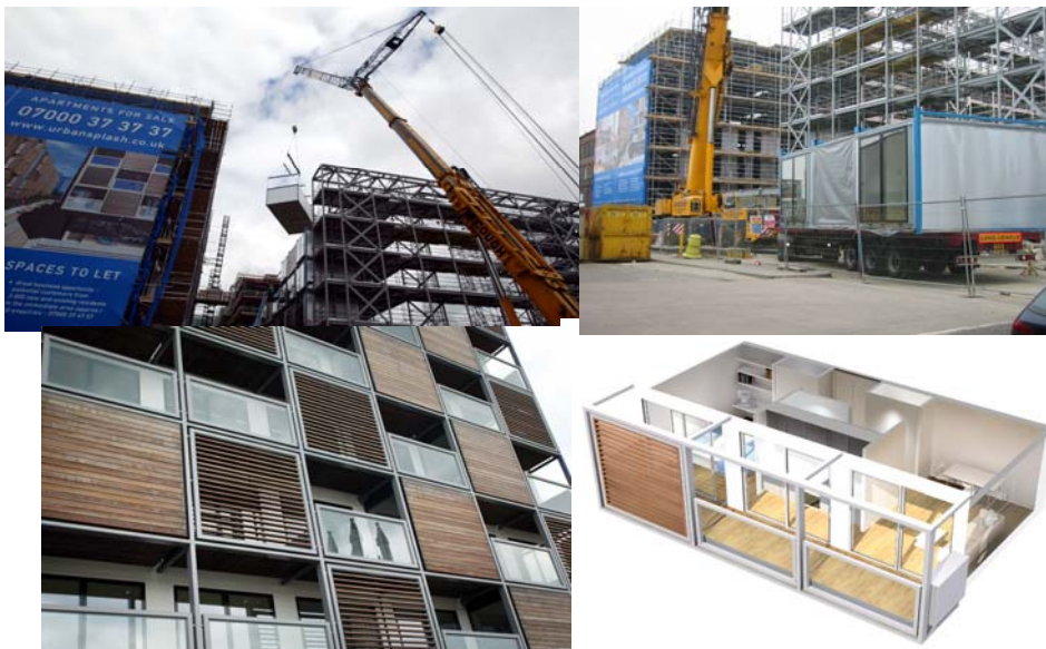
Steel 'Exo-Skeleton' with Modules Internally, Manchester
